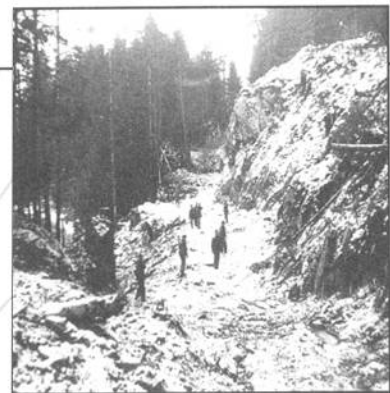
"A crew working to build road to top of mountain where station was built." Richard Pettinger
